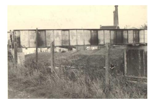
Circa 1962: the bridge's supports have been raised but the overhead lines have not yet been installed.
